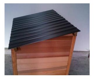
Step 18: Rivet ridge flashing to roof on every second rib, as shown.
