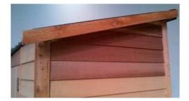
Step 23: Attach spouting channel to roof, riveting approx every second pan.
